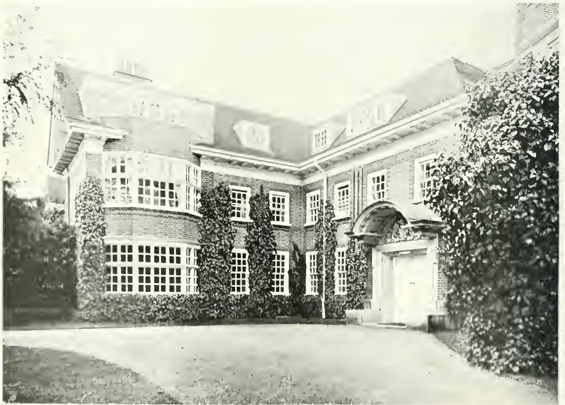
1313 HOUSE, ENGLAND. BUILT OF GREY BRICKS WITH RED BRICK FACINGS. THE HOUSE HAS A FIELD ROOF, A STONE DOORWAY, AND A CORNICE OF WOOD.
